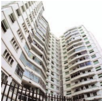
Figure 52 Immeuble Ecran Situation : Boulevard Bougara, 1959 (Piaton, 2016)
