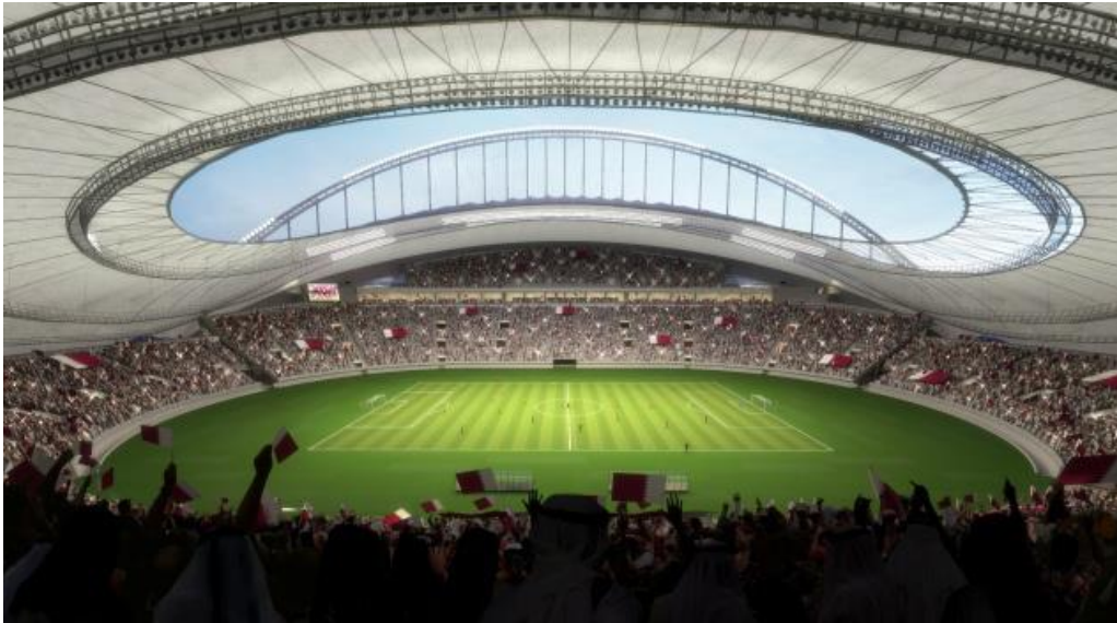
Figure II.46: View of the grandstand and the public bleachers of the Khalifa Sport City stadium (Qatar)
