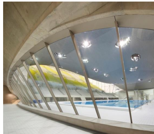
Figure II.65: Interior view of London Aquatic Center
