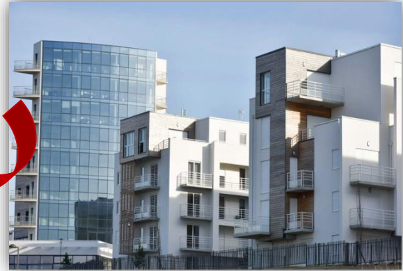
Figure 25 facade maritime. Source : www.ville-boulogne-sur-mer.fr
