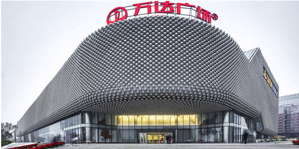
Figure 45 la façade principale du projet. Source: https://www.archdaily.com/463807/hanjie-wanda-square-unstudio
