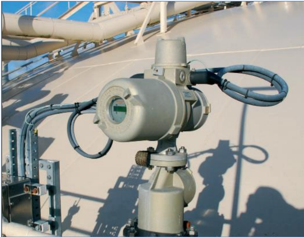
Figure I-7: Jaugeur asservi ENRAF. [6]
