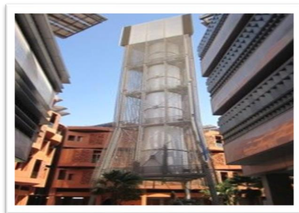
Figure 65: tour a vent Masdar city.
