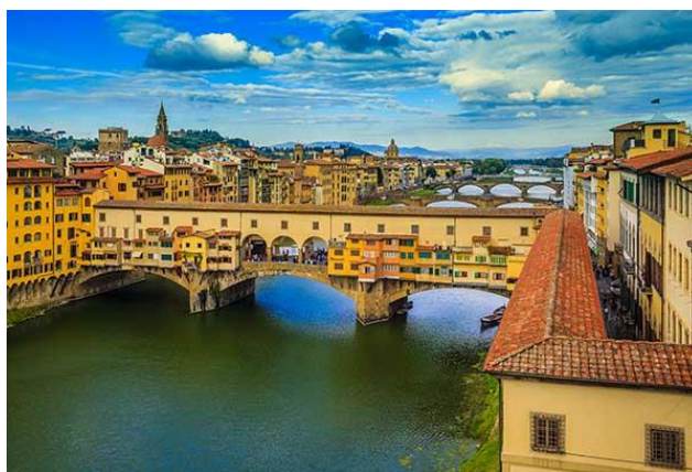
Figure 13: pont de vecchio de florence
