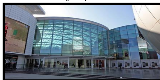
Figure 110: l'accès principal au mall. Source : https://www.google.com/url?sa=i&url=https%3A%2F%2Fwww.moroccomall.mall .
