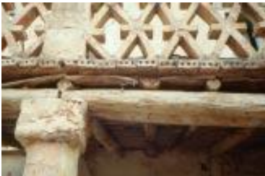
FIGURE 9: LE SYSTEME D'AERATION
