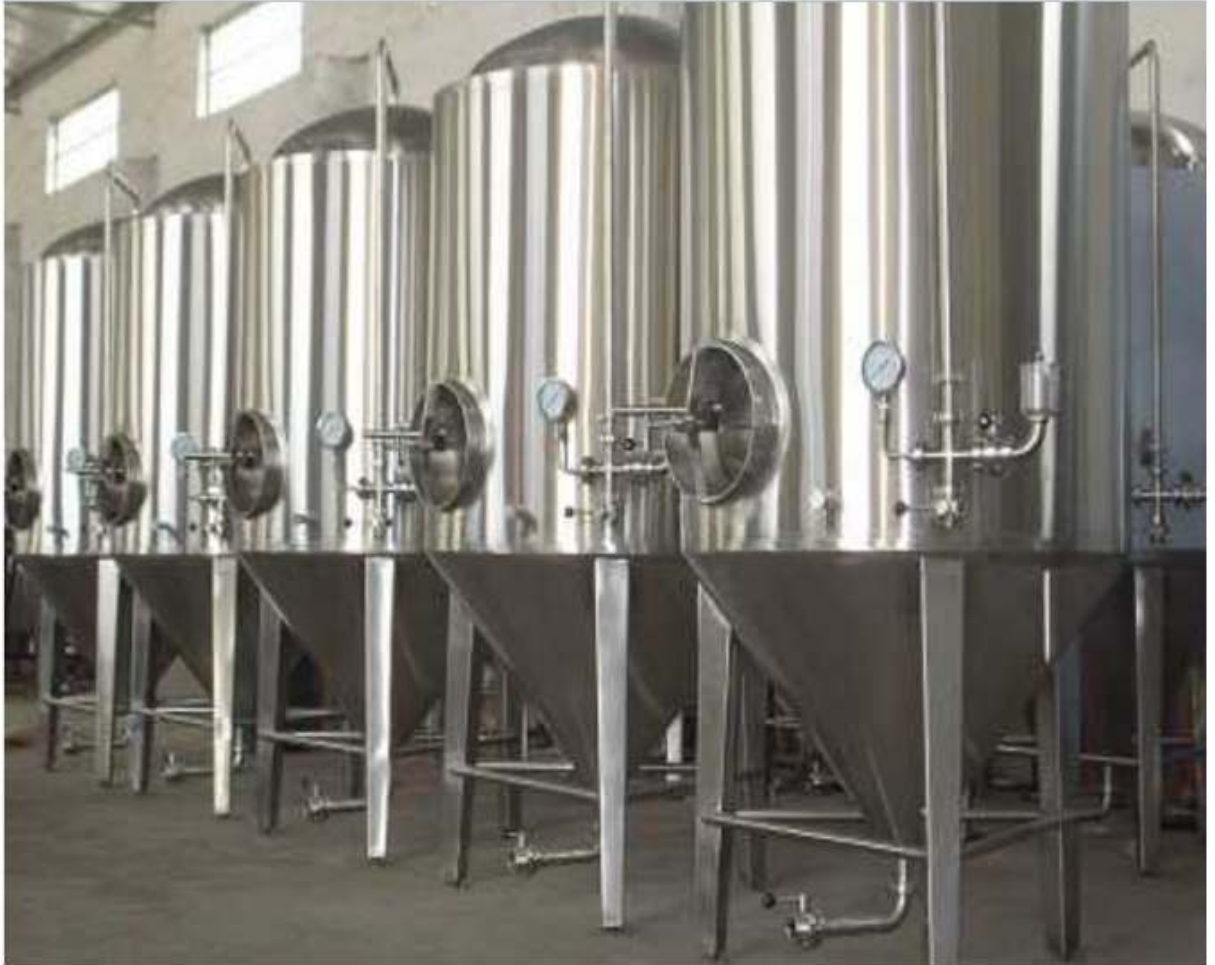
Figure 1.6: Les cuves de la station NEP.
