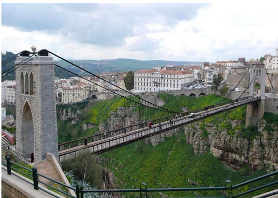
Figure 39: câbles de retenue, source : https://www.easyvoyage.com/photos/algerie/12233_consantine-1625
