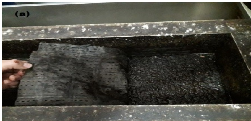
Figure IV.20 (a)- Placement de la nappe géogridle.
