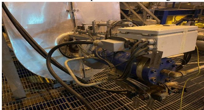
Figure I.9: vanne bypasse MP
