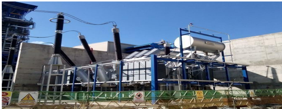
Figure I.6: Transformateur principal
