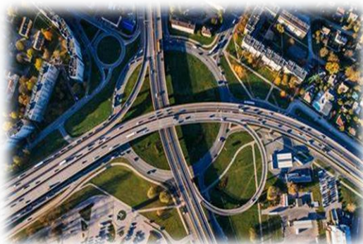
Figure 4 Infrastructure Source : 2Q== (300×168)
