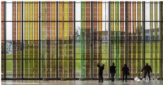
Figure 27:Brise-soleil Orientable Source : Laussane convention center 2025
