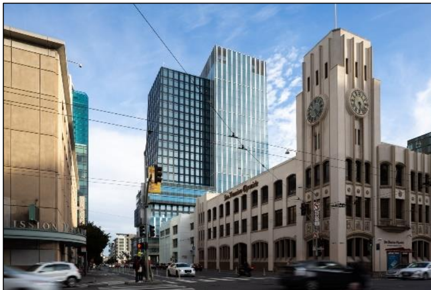
Figure 13: 5M Project Source: https://sfyimby.com
