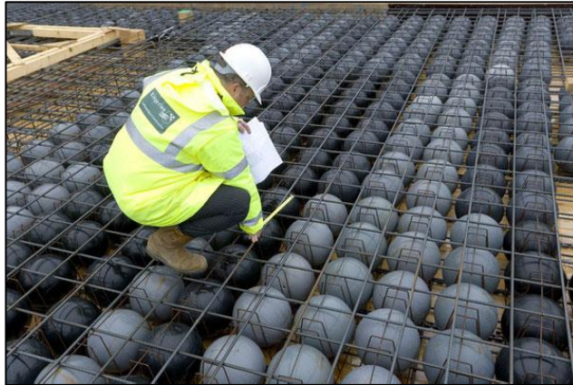
Figure 152 : Planchers cobiax Source : https://nouvelr-architecture.jimdofree.com/
