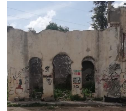
Figure 41: Façade Est. Source : Auteur, 2025.
