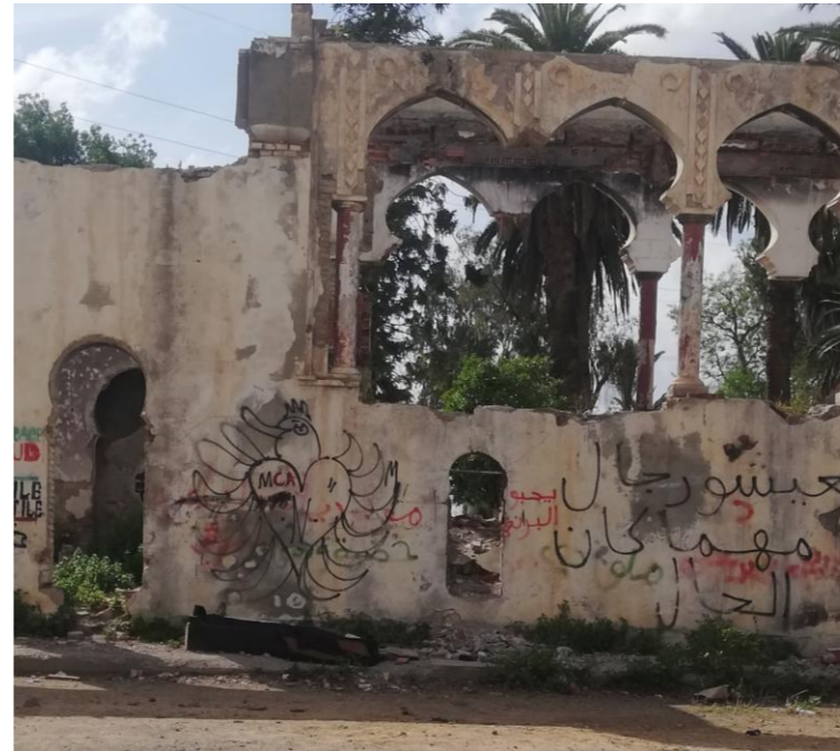
Figure 71: Ouverture façade Est.
