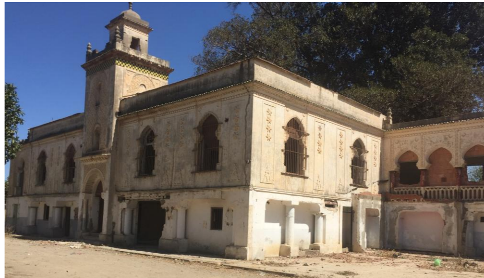
Figure 41: Façade Ouest. Source : BET Handassa wa bina, 2017.
