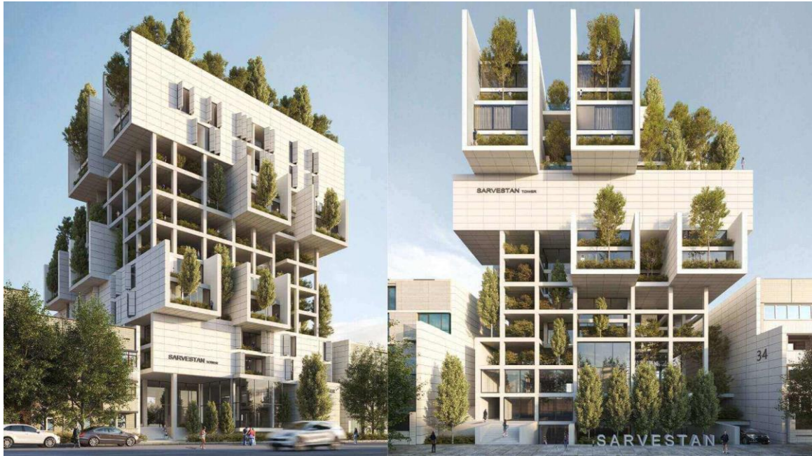
Figure 45 : Sarvestan Building à Iran. Source : www.amazingarchitecture.com
