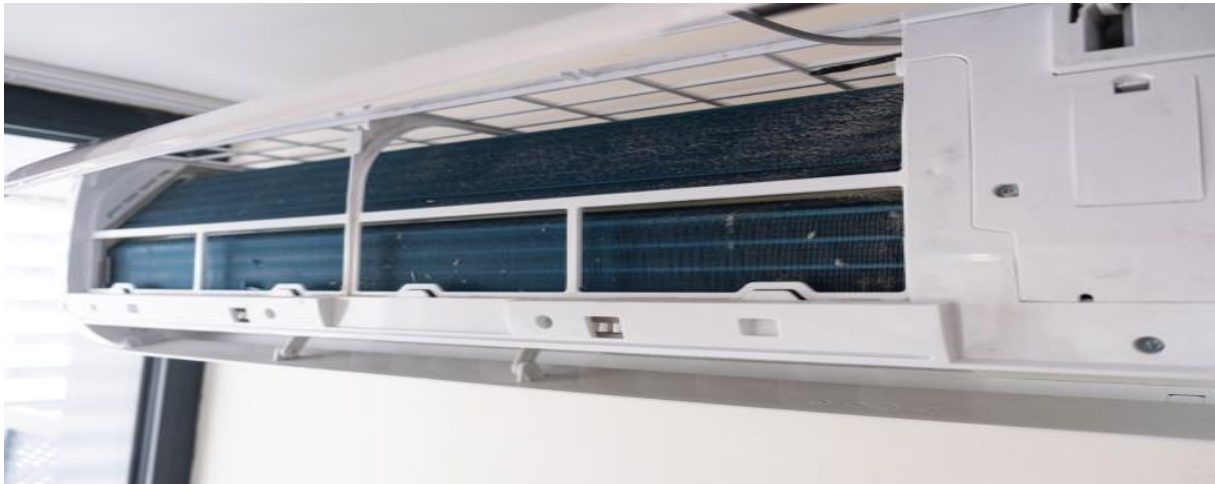
Figure 4: L'évaporateur [6]
