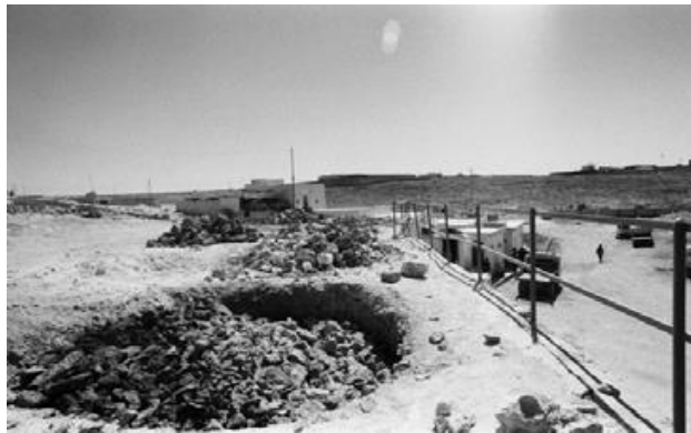
Figure36: Phase de construction
