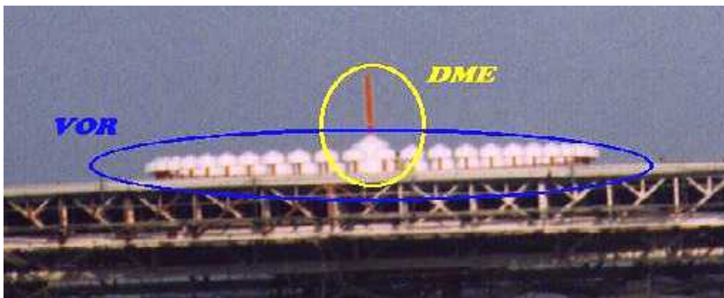
Figure 1.3 : Station VOR / DME.
