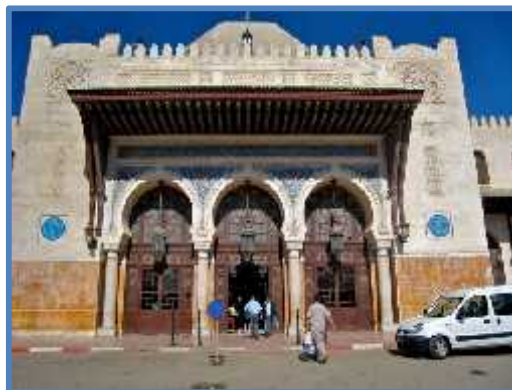
Figure 9 Façade principale Source http://www.oran-dz.com/economie/transports/gare-ferroviaire
