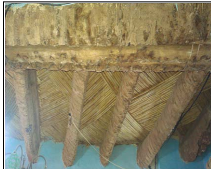
Fig.3.44 plancher a Roseaux
