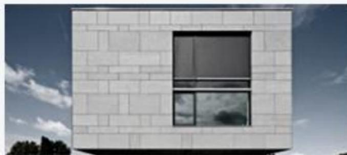
FIGURE: BARDAGE PANNEAU FIBROCIMENT
