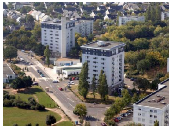
Figure 25 : Photo de batiment, Source :Lacaton & vassal.
