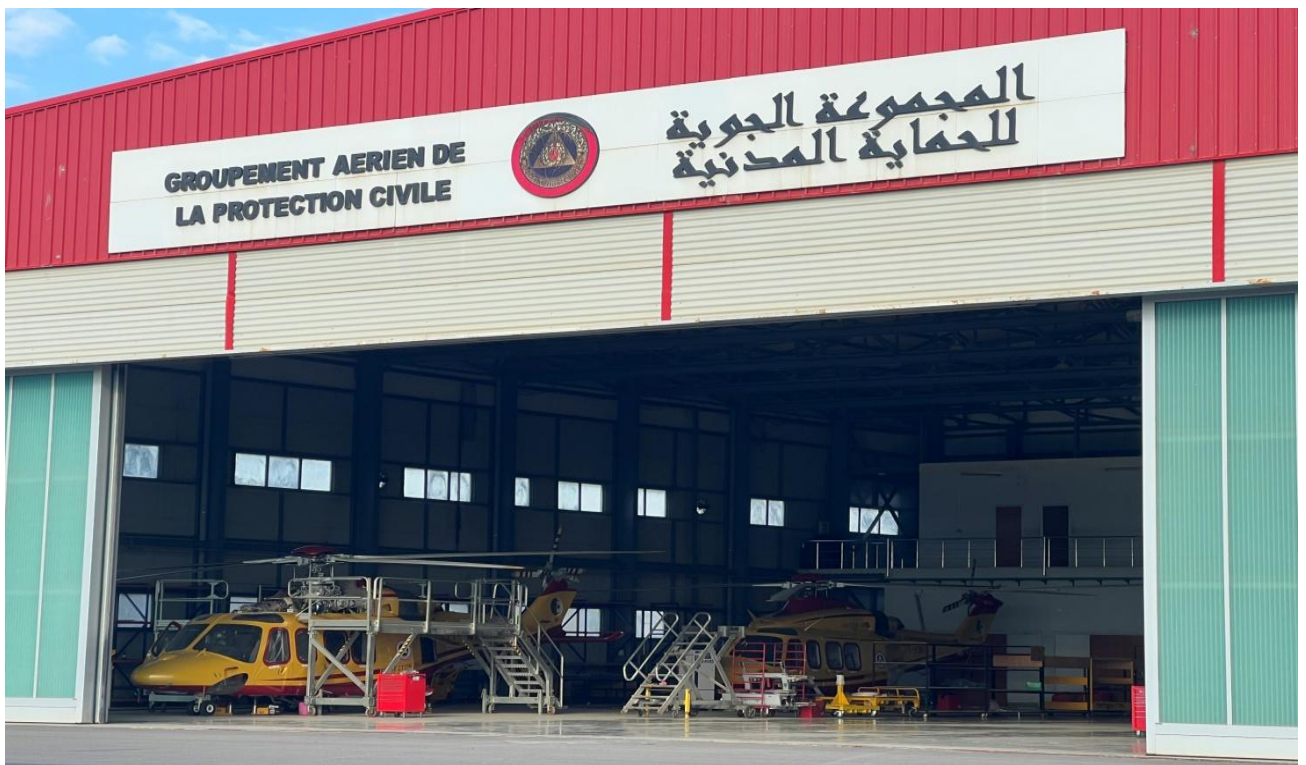
Figure 2.1: The Civil Protection Air Group hangar
