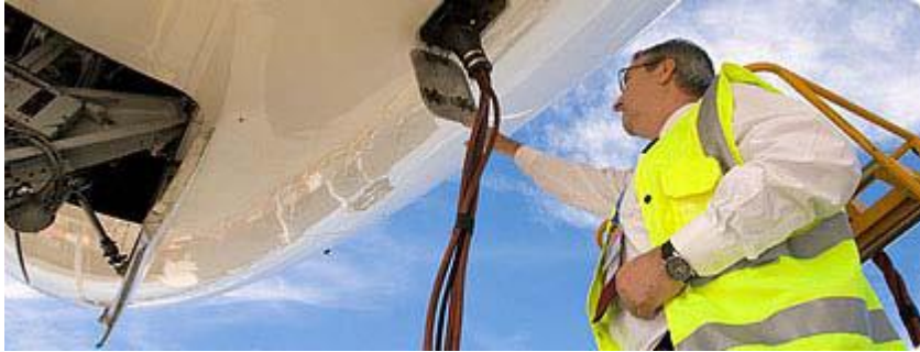
Figure4.4: Example use of FEGP at Stansted airport[17]
