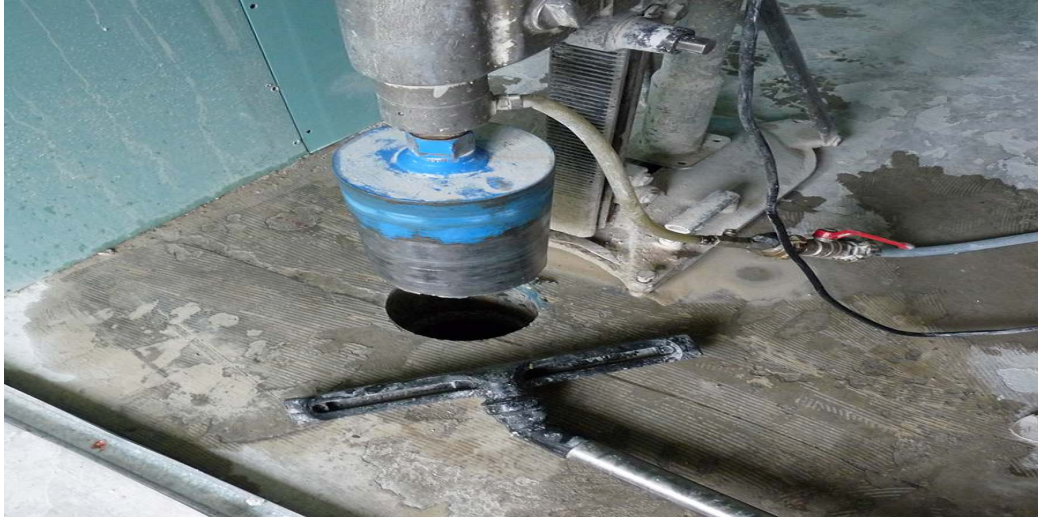
Figure I.19: Carottage.
