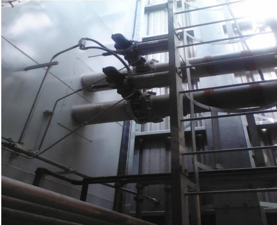
Figure I-9: Vannes anti-pompage
