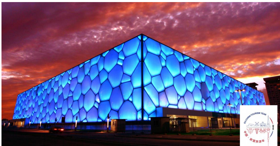
figure 50 : Photo du Water Cube, Source : https://ecty2018.org/the-water-cube2/
