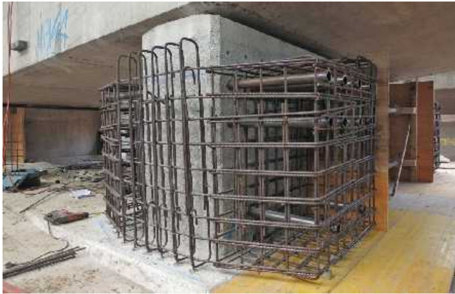
Figure I-53 : Technique de chemisage [2]
