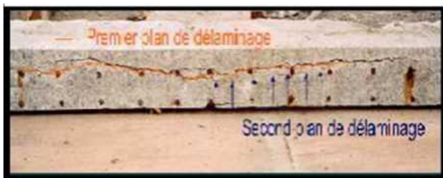
Figure I-43 : délamination [5]
