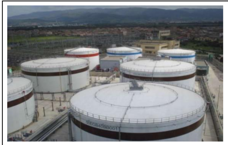
Figure 1.6 Station de carburant.
