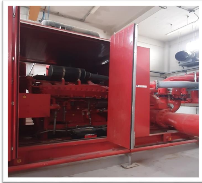
Figure 2.4 pompe diesel.
