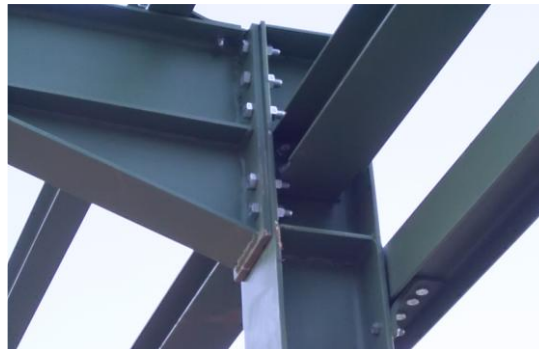
Figure1.7.1: Bolted connection
