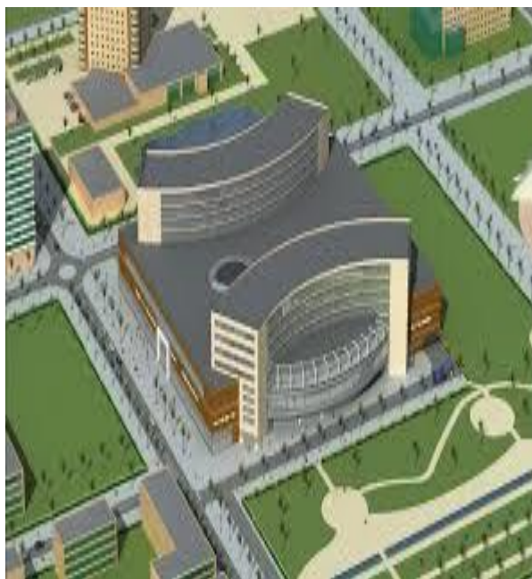
- Figure 11 : centre commercial de Bab Ezzouar
