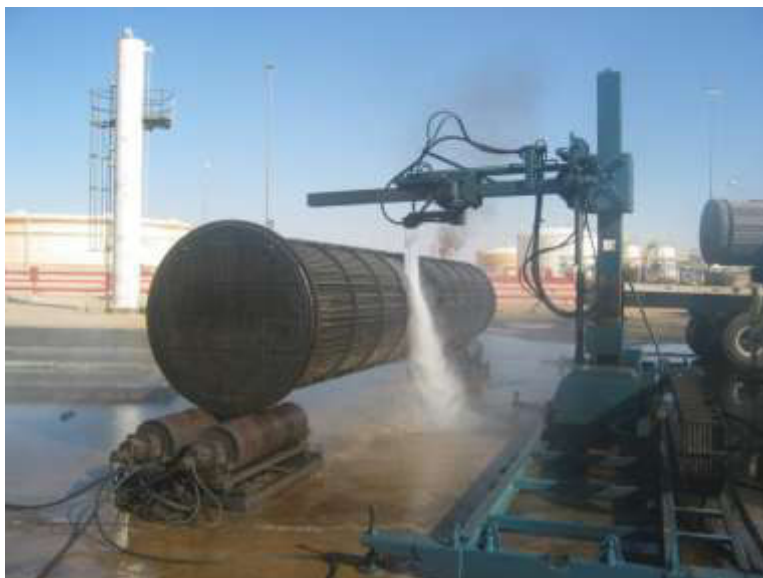
Figure (III.34) : nettoyage hydraulique.
