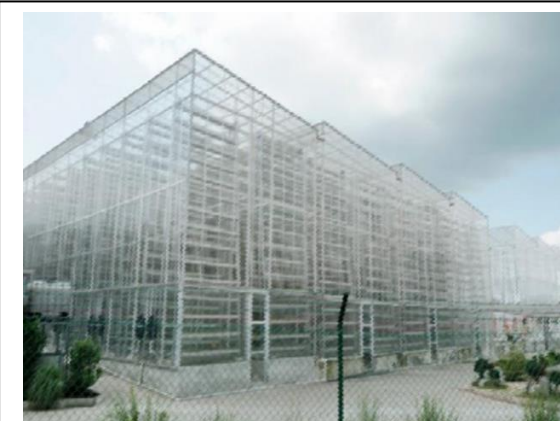
Photo 01:Serre Sky Green Source : http://www.transition-verte.com/singapour-une-windowfarm-geante/
