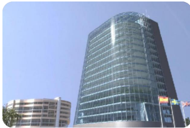
Photo 1 :Bâtiment Plontagon Source : http://plantagon.com/urban-agriculture/vertical-greenhouse/integrated
