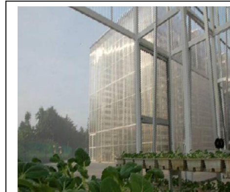
Photo 02 :Serre Sky Green Source : http://www.transition-verte.com/singapour-une-windowfarm-geante/
