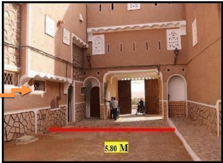
Figure 3.31 Photo : voie secondaire/source:www.Tafilelt.com
