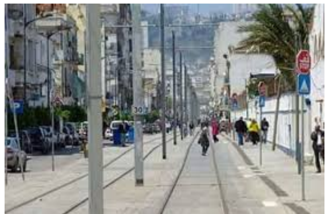
Figure 2.20: Photo Tramway Avenue Tripoli (Source web: Google Image)
