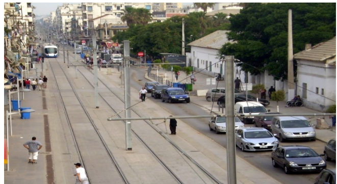
Figure 2.22: Photo Tramway Avenue Tripoli (Source web: Google Image)
