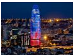
Figure 79 : Torre Agbar Barcelona
