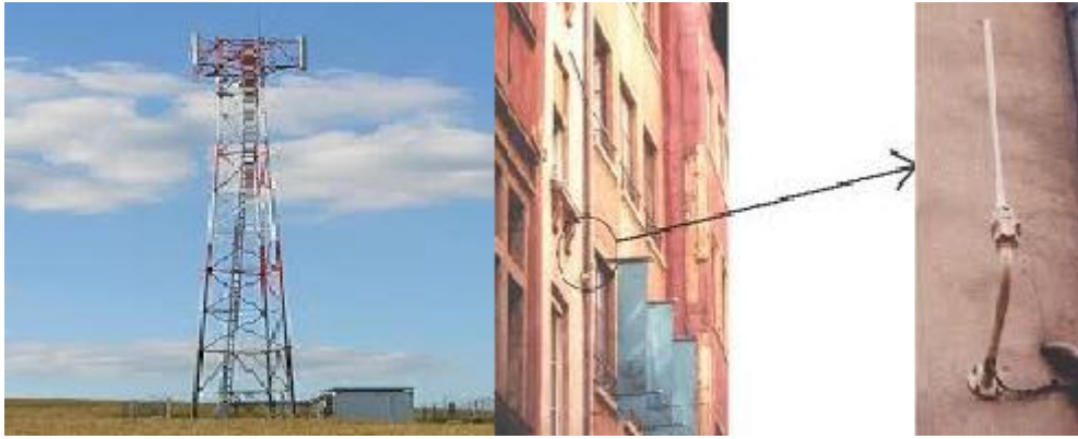
Figure 1- 2: Exemples des BTS (BTS normale et micro BTS)
