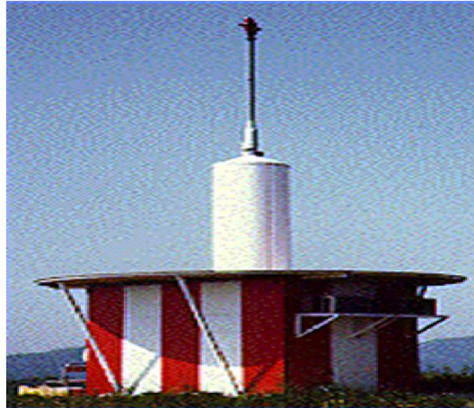
Figure 1.2 : Station VOR / DME.
