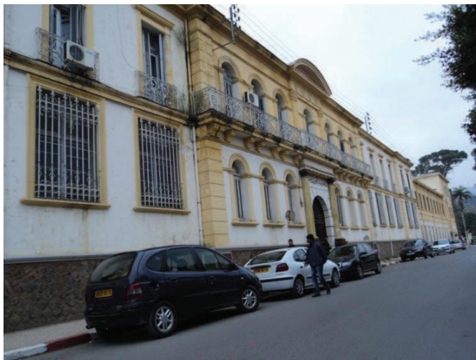
Figure.1.9 Lycée Ibn Rochd (Epoque Coloniale)
