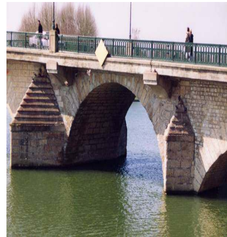
Figure 3.4: Le pont de Joigny (France).
