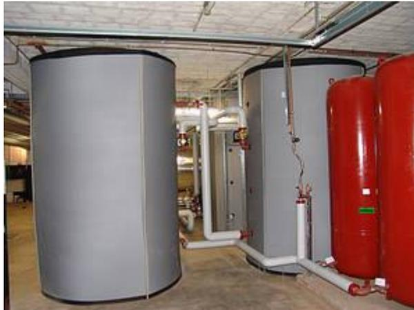
Figure 3.6 : Cuves de stockage [34]
