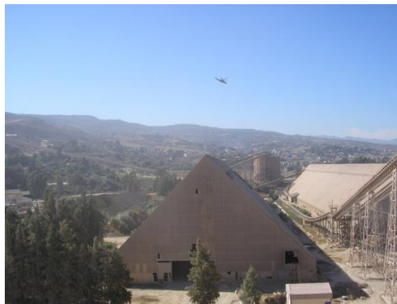
Figure 1.10- Halls de stockage [1].
