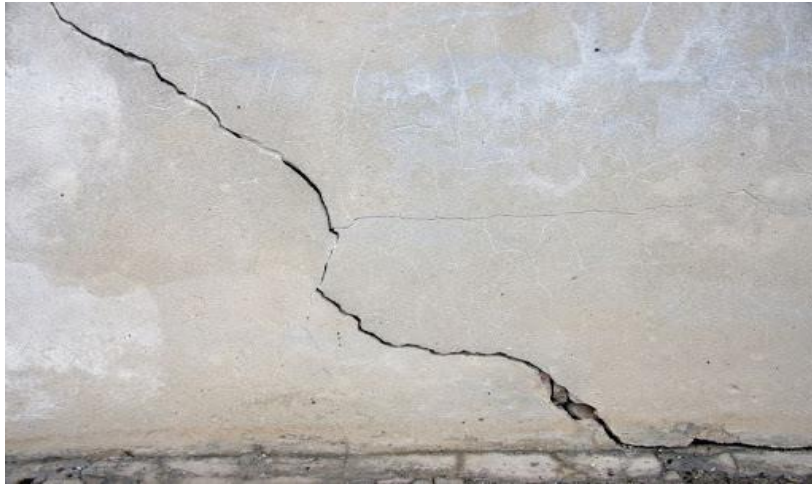
Figure I.7 : fissuration
