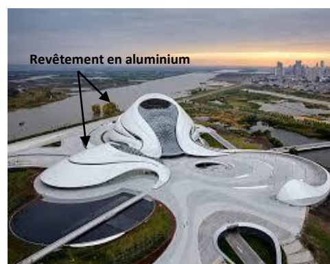
Figure 78 : Façade Harbin opéra house. Source : www.japan-architects.com
