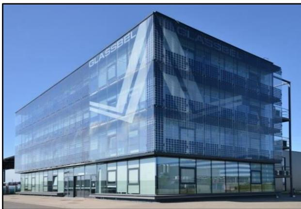
Figure 12 : Le verre photovoltaïque Source : [https://www.researchgate.net/figure/SmartFlex-modules-wwwsmartflex-solarfacadeseu-project-Source-SUPSI-modules\\_fig15\\_332556585](https://www.researchgate.net/figure/SmartFlex-modules-wwwsmartflex-solarfacadeseu-project-Source-SUPSI-modules_fig15_332556585)
