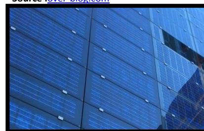
Figure : façade photovoltaïque
