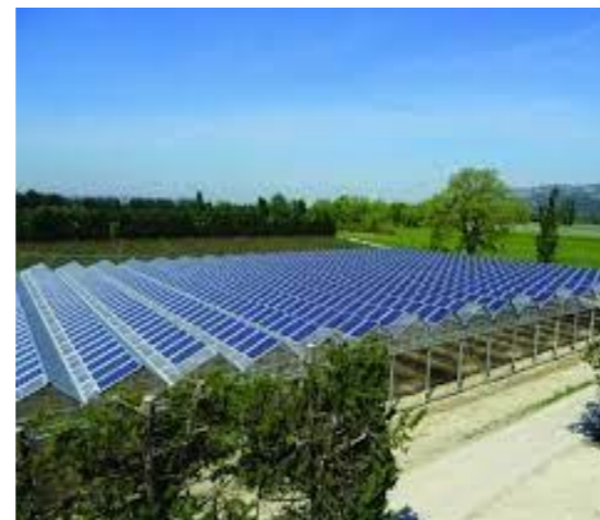
Serre agricole photovoltaïque Source : https://www.batimentphotovoltaïque
