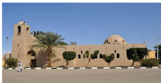
FIGURE 3 : LA MOSQUEE DE GOURNA SOURCE : HTTPS://WMF.ORG/
