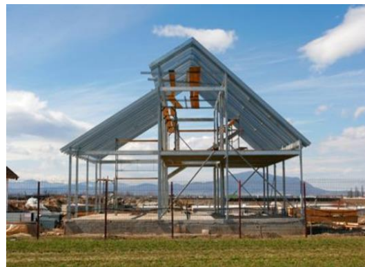
FIGURE II.5: STRUCTURE EN ACIER
